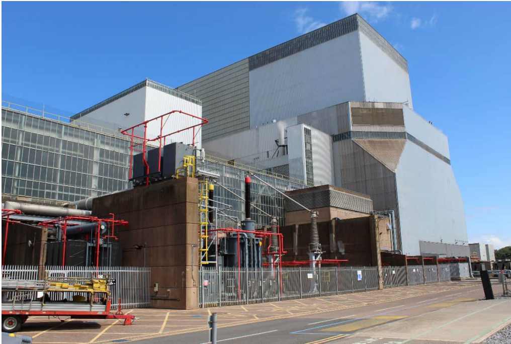
Plate 1. The original turbine hall and reactor building. View north-east.
