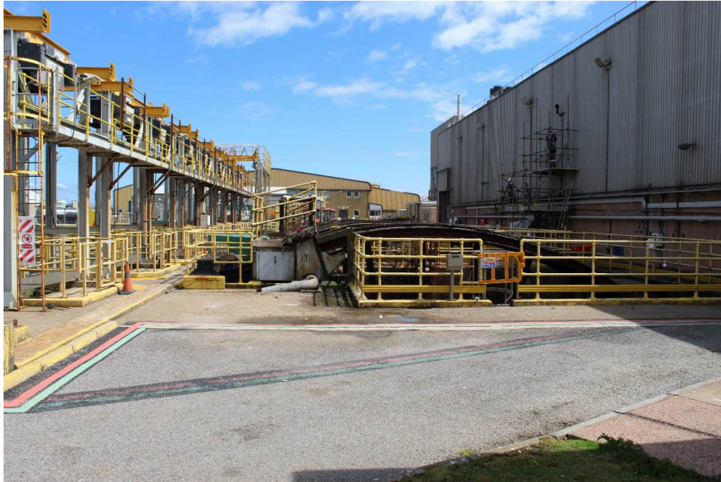
Plate 13. Pumphouse in the northern site area. View east.
