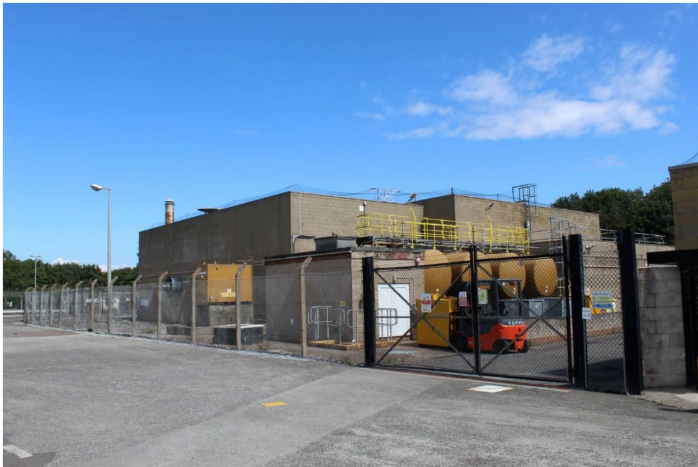
Plate 8. Original ancillary building in the eastern site area. View north-east.
