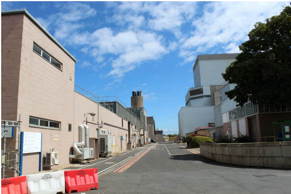
Plate 12. Original workshop buildings in the northern area of the Site. View east.
