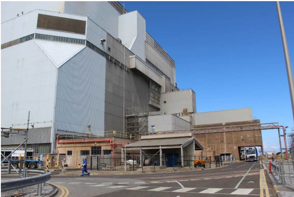
Plate 2. The reactor building. View north-west.
