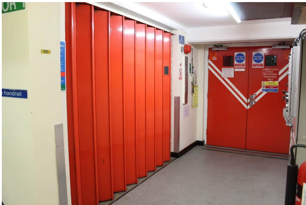
Plate 18. Reactor building interior features.
