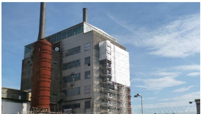
Figure 6. Reactor one cladding and glazing work
