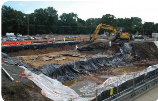
Soil is Excavated and Covered with Plastic Tarps 1
