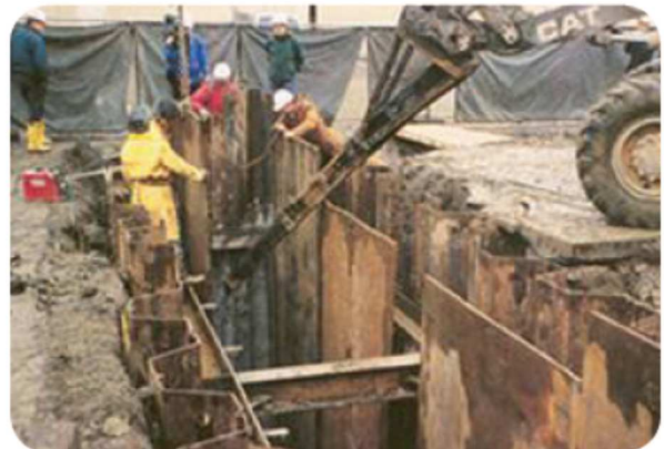
Construction of a Permeable Reactive Barrier 1
