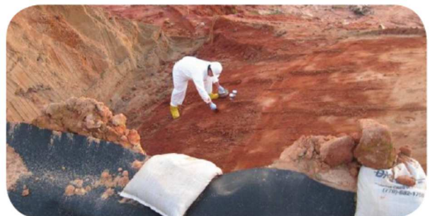
Worker Collects Soil Samples to Verify Site is Clean 1
